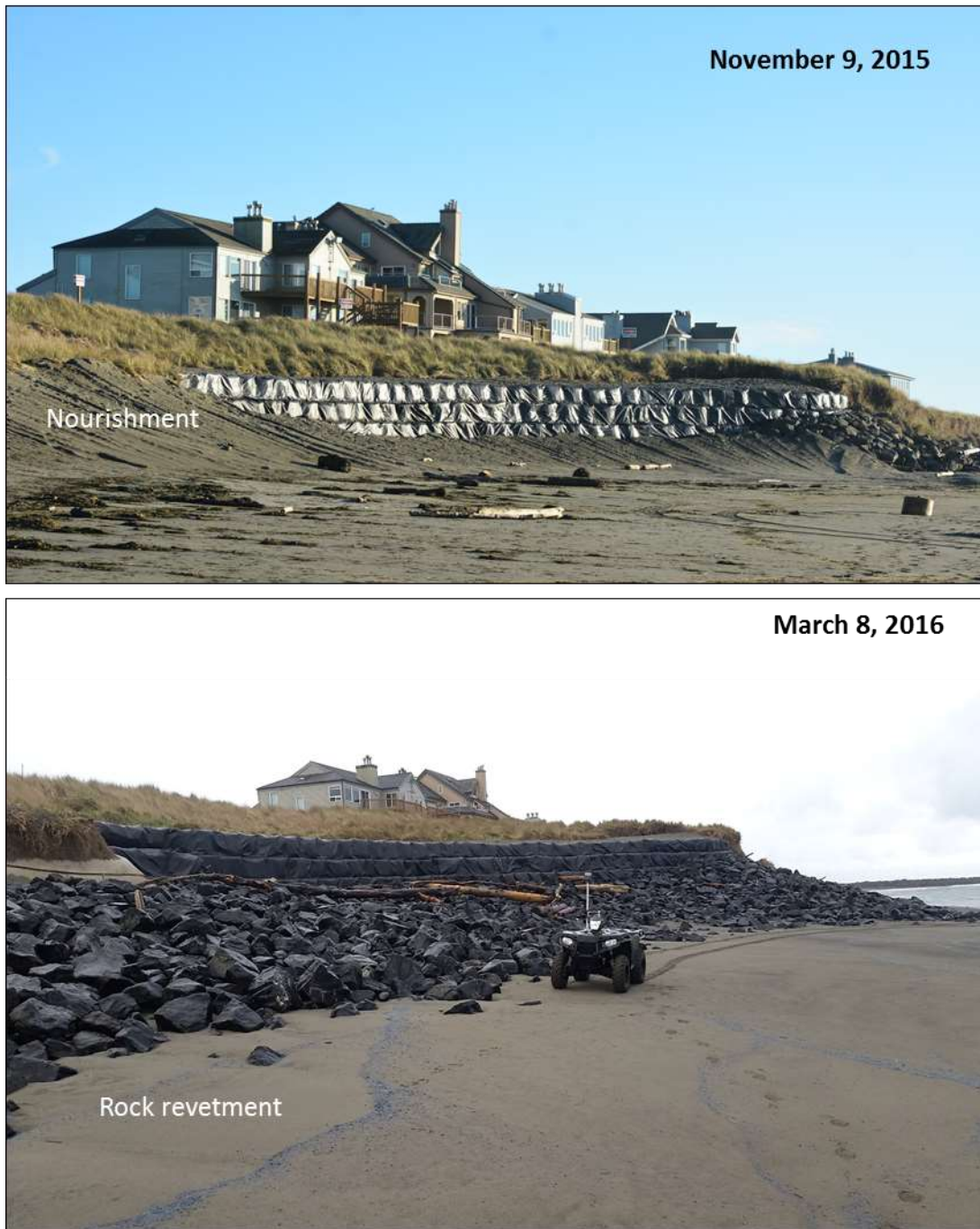
Figure 8-19 Geobags Nov. 2015 and Rock Revetment Installed in Front of Geobags Winter 2016
