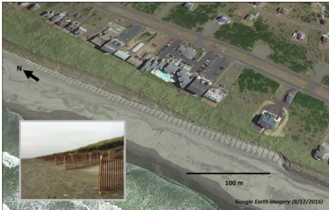
Figure 8-21 Sand Fences Installed North of the Ocean Shores Rock Revetment in 2016
