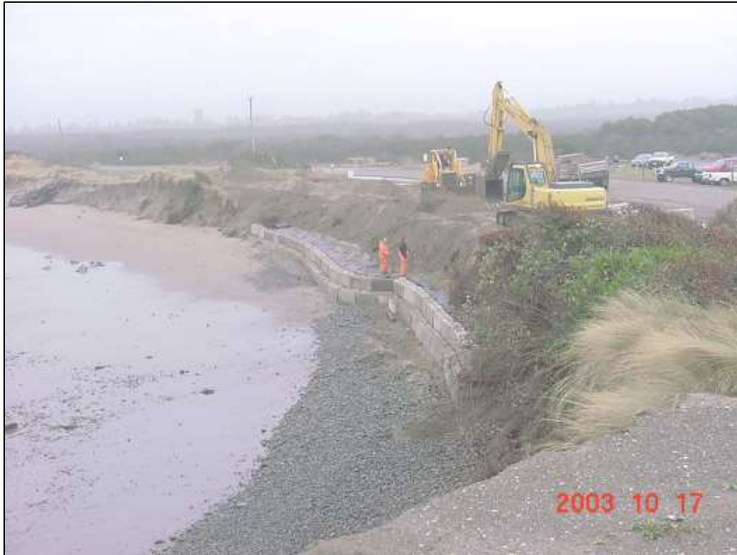
Figure 8-10 Emergency Dune Protection Constructed at Half Moon Bay, Westport, October 2003
