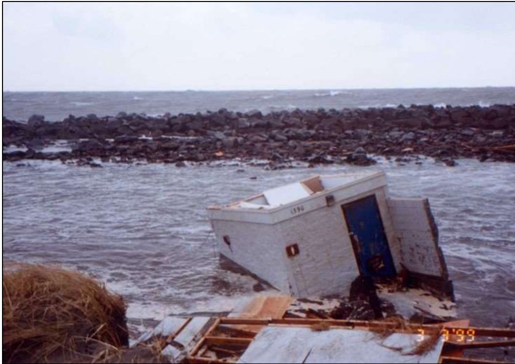
Figure 8-15 Flooding and Erosion of the Ocean Shores Public Restroom During March 1999 Storm
