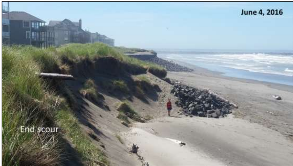
Figure 8-20 Eend Scour North of the Ocean Shores Rock Revetment
