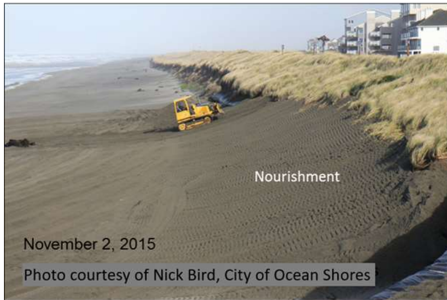
Figure 8-18 Photos of Geobags and Dune Nourishment at Ocean Shores in November 2015
