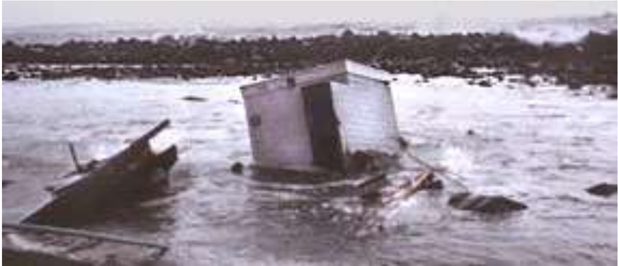
Figure 11-18 Restroom at North Beach Destroyed by Winter Storm Waves
