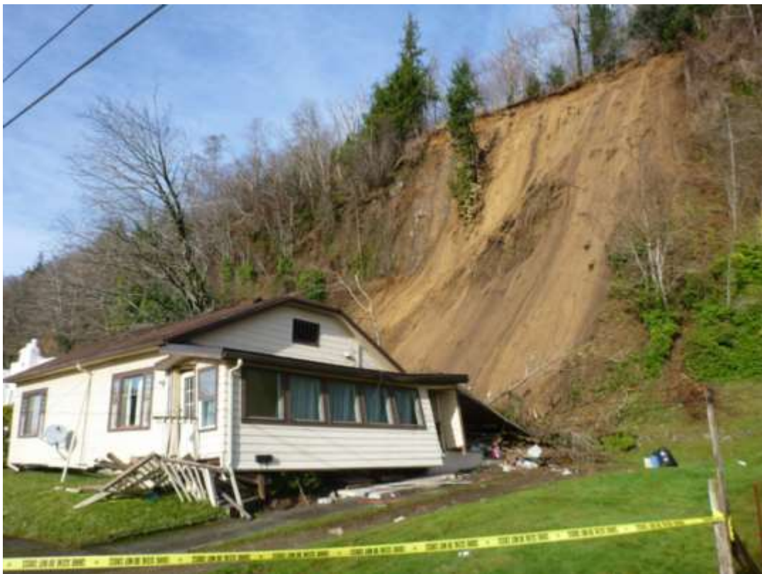
Figure 10-7 Structure Impacted by January 2015 Landslide Event
