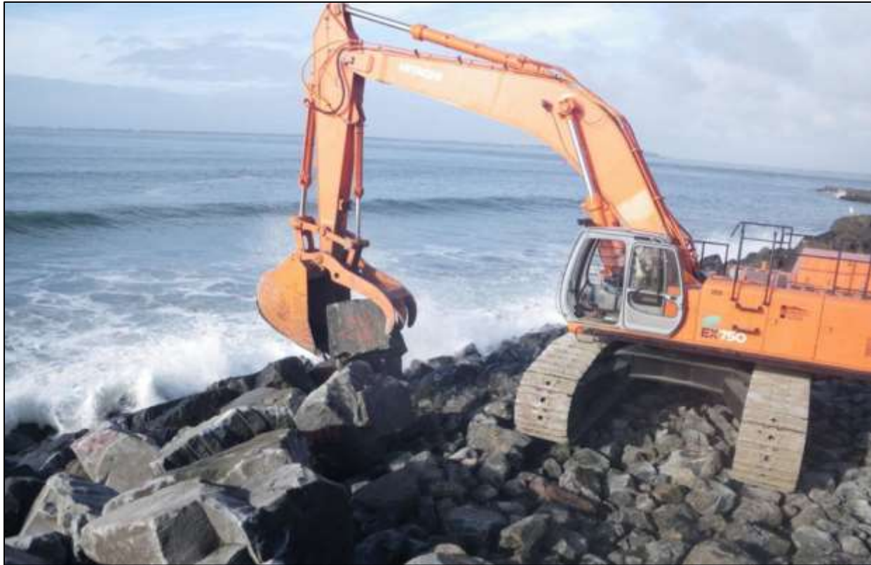
Figure 8-12 Photo of Point Chehalis Revetment Repairs in 2013 from Michalsen and Brown (2015)
